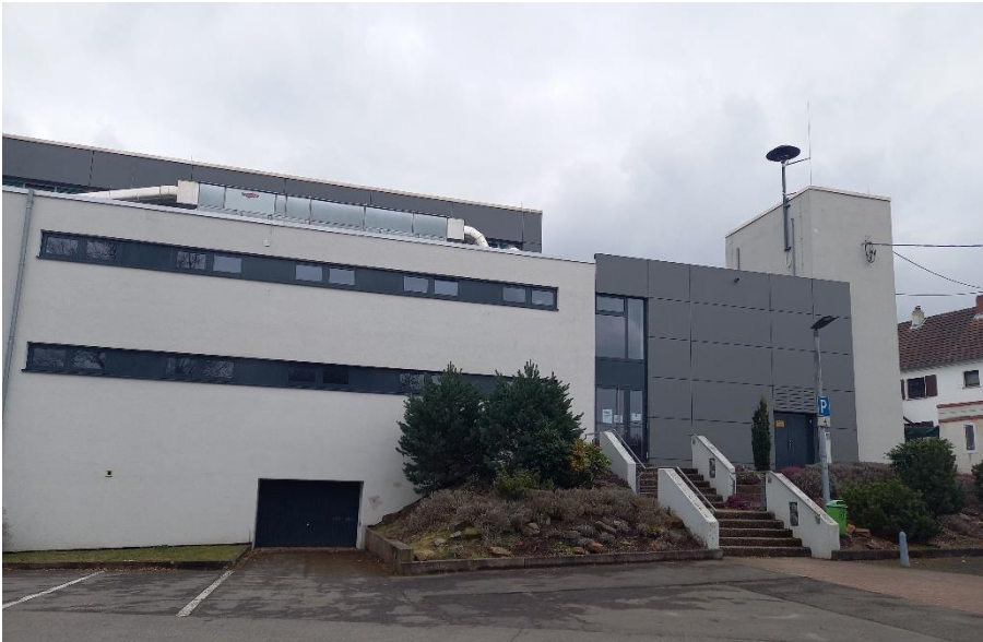
Abbildung 36: Ostertalhalle in Hangard
